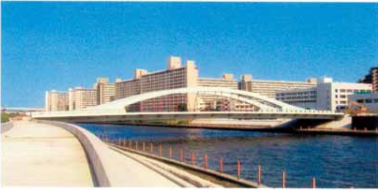
Fig.1 The Shin-Toyo Bridge (Steel box girder bridge with CFT arch ribs)
